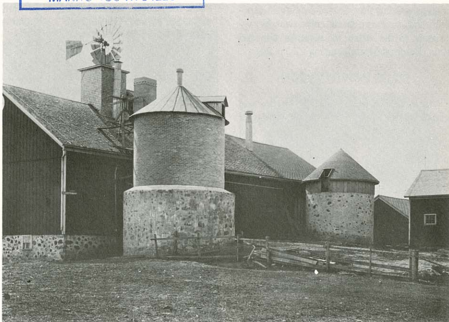
1910 photo of silos on Louis Wiegand farm in Centerville. Fieldstone silo in rear was built in 1900, and may be the oldest in Manitowoc County. Note chimney on brick silo (1910) which may have been used for ventilation or heating. Both in excellent condition today.
