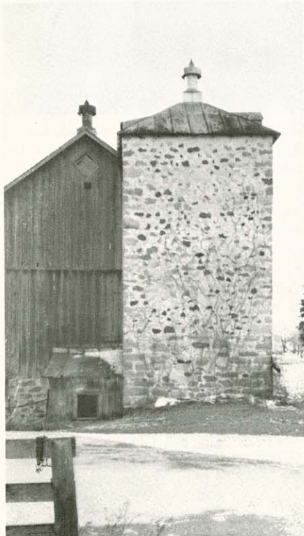
Fieldstone square silo built in 1933 from old stone fence and other stone on Bill Christel farm south of St. Nazianz. Bill, 80, and neighbors built it themselves with muscle and sweat.
