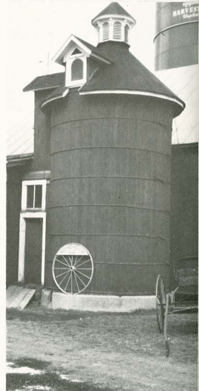
Wood stave silo on Roy Schmidt farm north of Two Rivers. Now part of Farm Museum.
