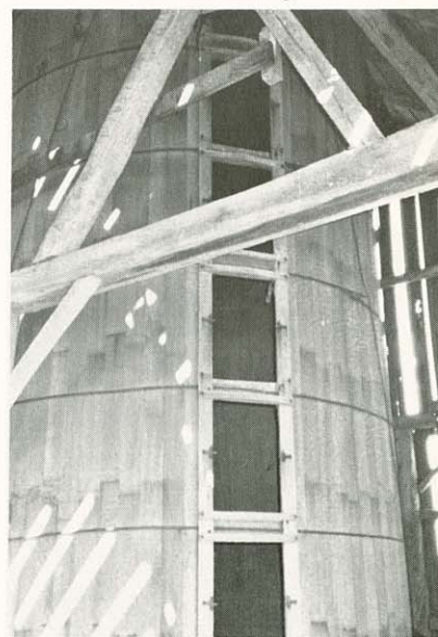
Sunlight peeking in on a round wood stave silo, inside the barn at the Vernon Schreiber farm north of Two Rivers. Silo doors were removed as silage level was lowered.
