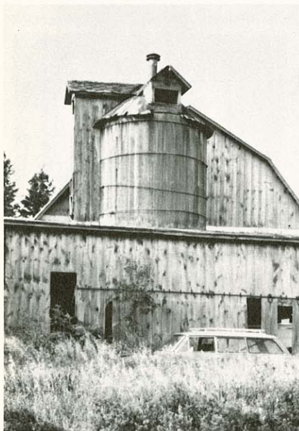
Wooden silo complete with wooden roof, filling hole, chute and vent pipe at Highway K and I-43 east of Kellnersville.
