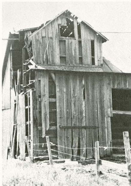
Square wooden silo built into the southeast corner of the Willis Voss barn, Town of Centerville. Most common type of the original silos built in Wisconsin.
