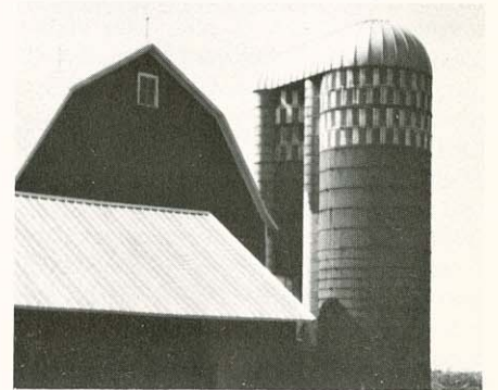
Example of twin silos with a common roof and top unloader. When one silo is empty, the unloader is raised and transferred into the other silo. Concrete stave type built in the late 1950's. Harvey Guse farm, west of Maribel.
