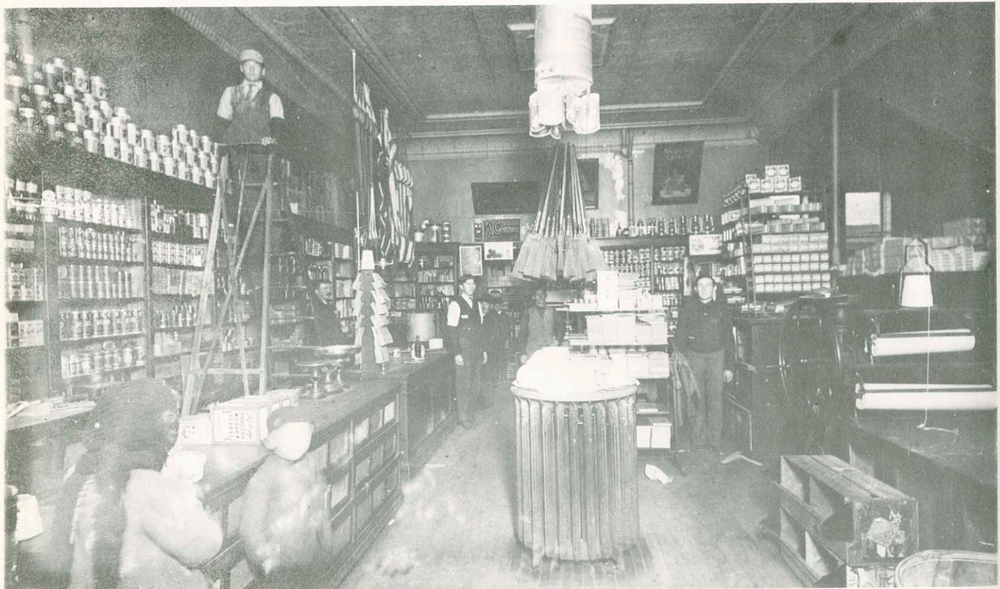
The grocery section before the 1916 addition.
